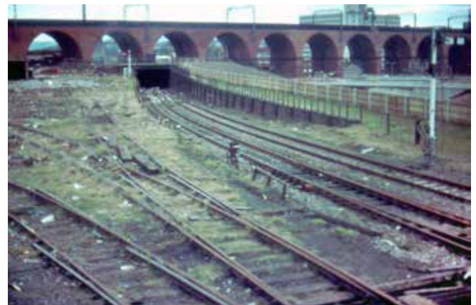
The west end of Wellington Road tunnel in April 1982. The tunnel ran from the George Road sidings seen on the left and under the LNWR main line on the viaduct.
